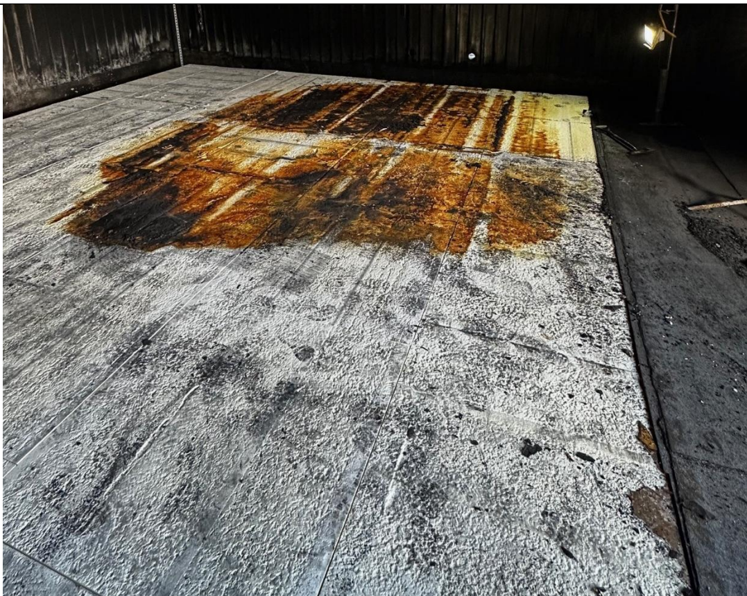
Figure 27: PIR insulation Post-test.
