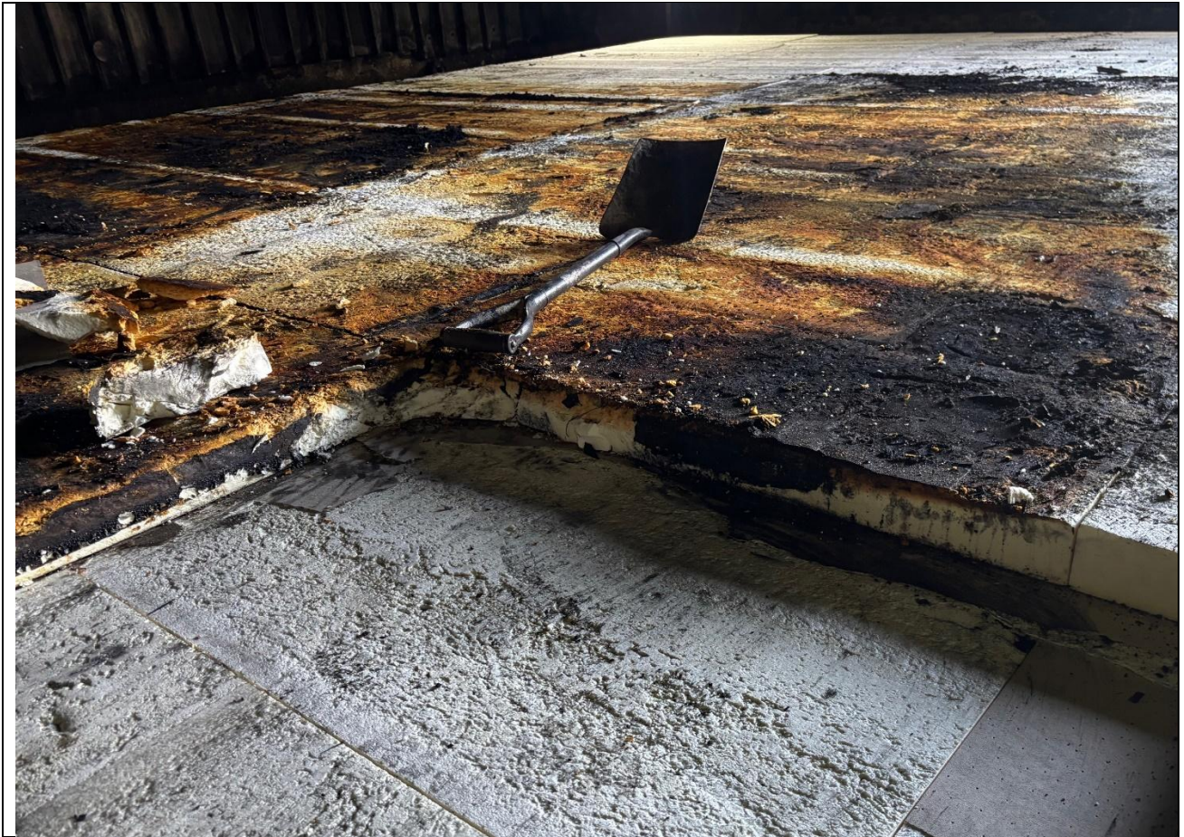
Figure 28: Charring depth within the PIR insulation Post-test
