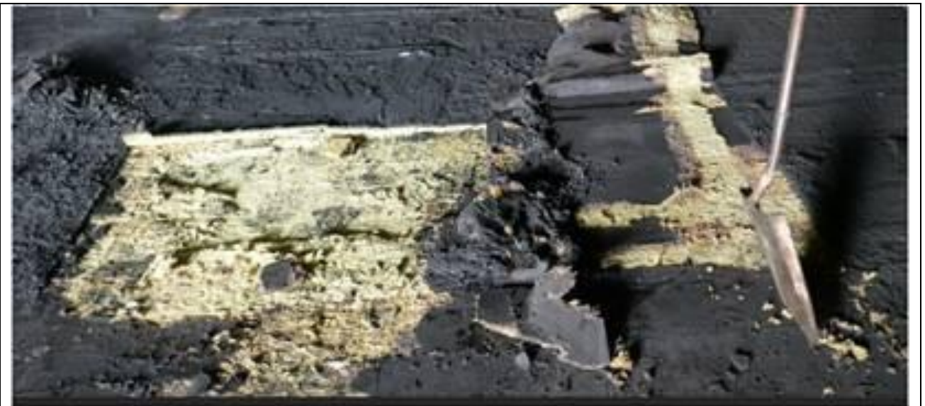
Figure 50: Charring depth within the Stone wool insulation Post-test
