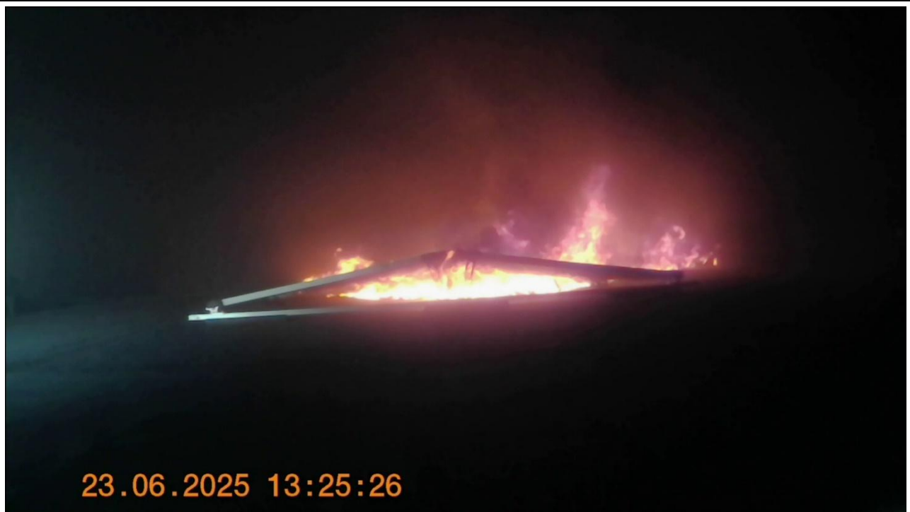
Figure 18: Fire begins to spread across roof assembly (Camera 3)
