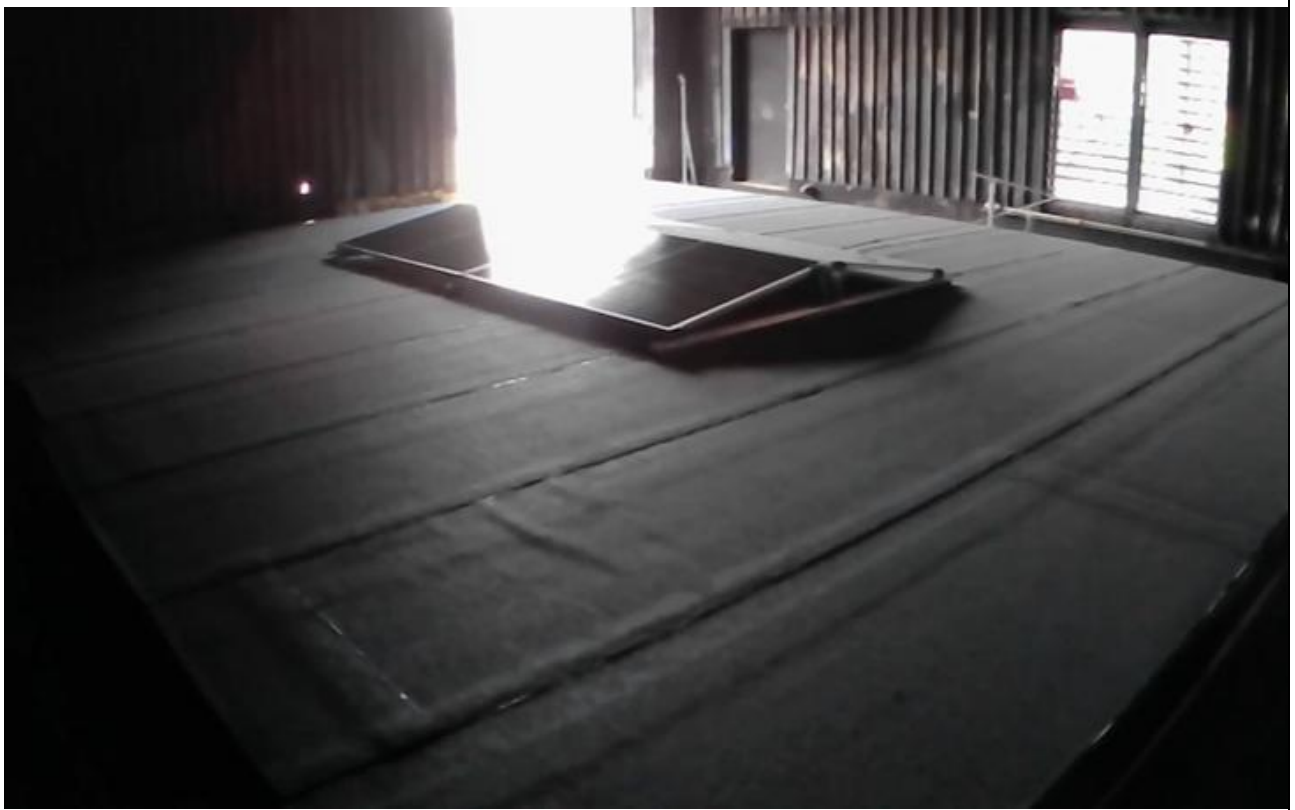
Figure 12: Video camera view back right corner of the roller shutter. (Camera 2)
