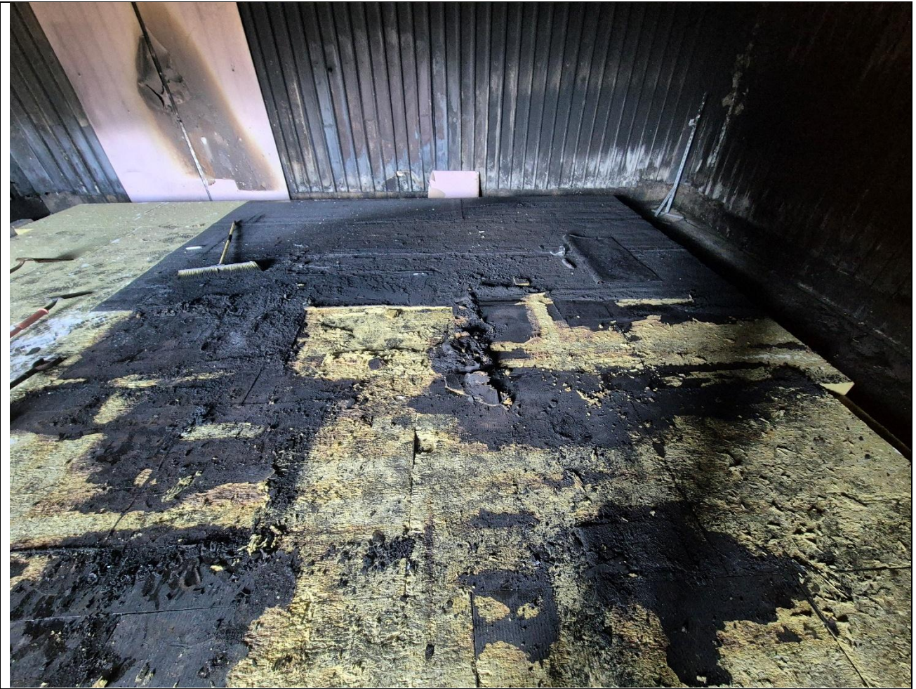
Figure 49: Stone wool insulation Roof Assembly Post-test
