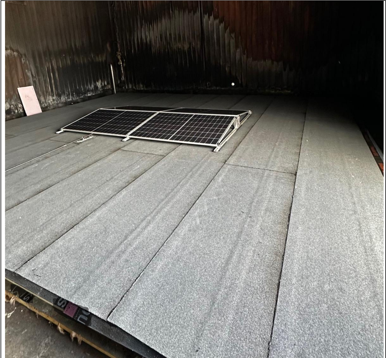
Figure 1: PIR insulation test roof assembly and set-up of solar panels.
