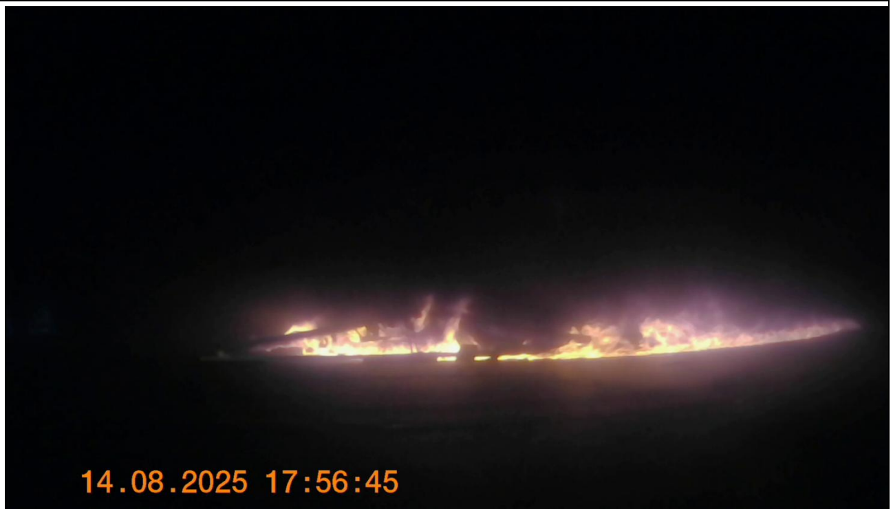
Figure 44: Fire exhibits further spread across roof assembly (Camera 3)
