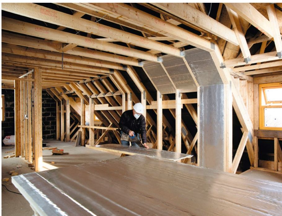
Simon says PIR/PUR insulation helps to create a well-insulated building envelope, reducing the need for heating and cooling systems.
