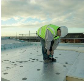
space possible. With lambda values as low as 0.021 W/mK, PIR insulation performance can be achieved with less thickness than other commonly used insulation materials. Its exceptional insulating properties, high strength and light weight, has seen it used across residential, commercial and refurbishment projects. It also has excellent water-resistance properties, making it suitable for flood risk areas.
