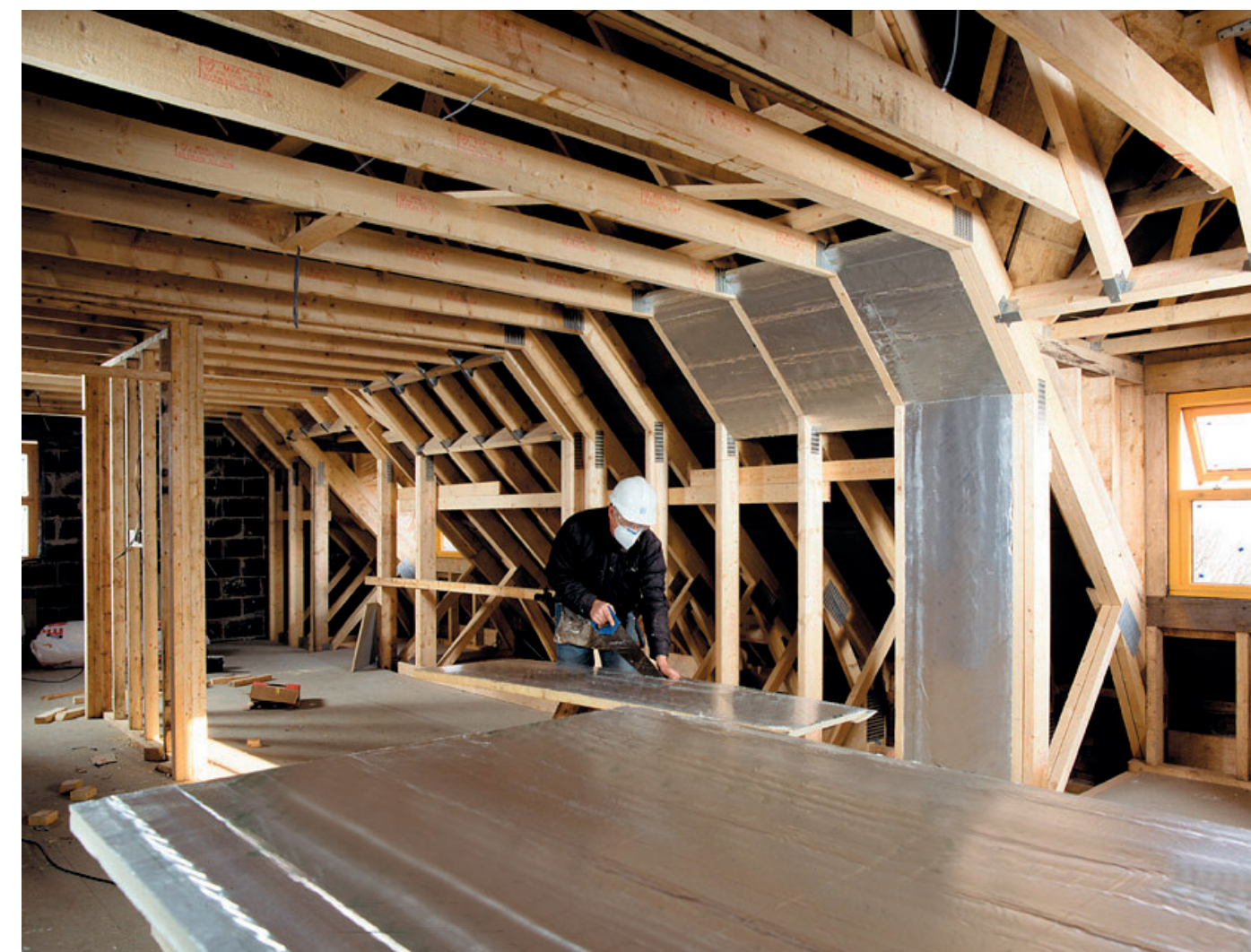
Above: Roof installation of PIR Boards; Left: Flat roof boards being installed: “To achieve more thermally-efficient building envelopes we must have a fabric-first approach.”
