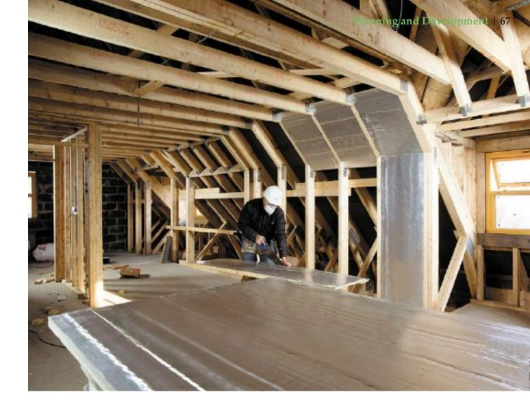
lambda values as low as 0.021 W/mK, PIR insulation performance can be achieved with less thickness than other commonly used insulation materials. Its exceptional insulating properties, high strength and light weight means it is used widely across residential, commercial and refurbishment projects.
